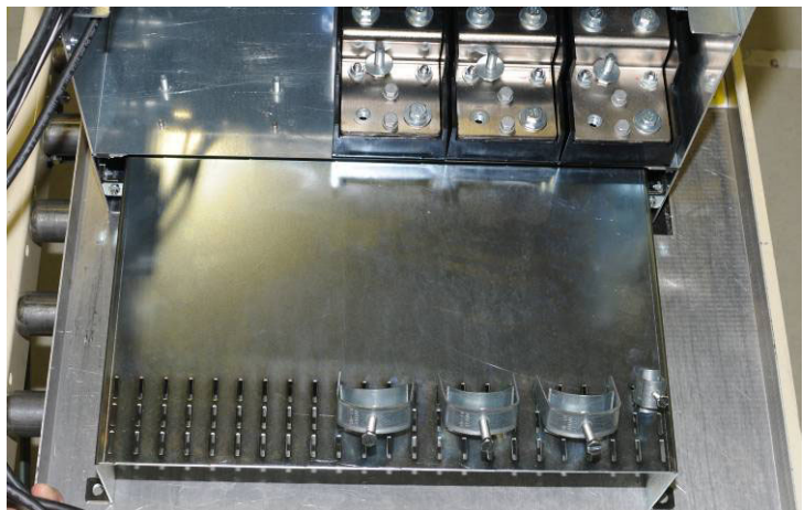
Figure 11. Cable-clamp bracket mounted on E2 frame.
